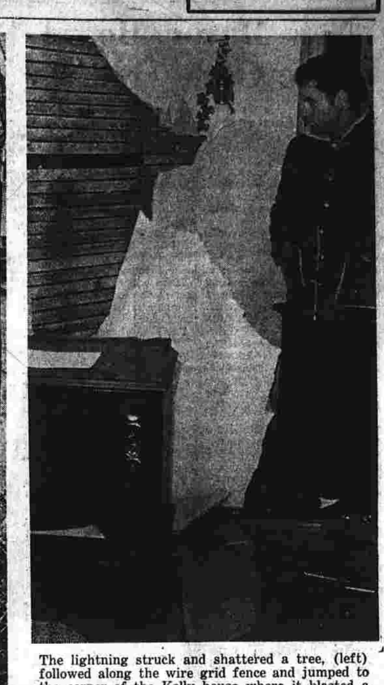
The lightning struck and shattered a tree, (left) followed along the wire grid fence and jumped to the corner of the Kelly house where it blasted a hole.
